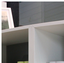
Carcass mitered tightly glued
